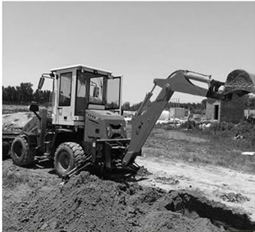
digging the ditch
